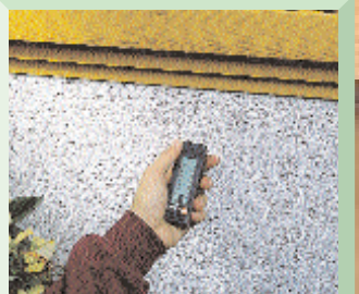
Measuring moisture distribution
